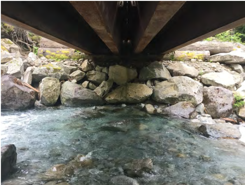
Left Bank Abutment when facing downstream
