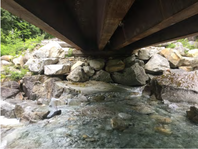
Right Bank Abutment when facing downstream
